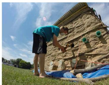
Our projected solution to the problem entails creating small vents in the wall near the base of the structure and on an adjacent wall near the roof. This is not culturally invasive and using the positioning of the vents to control air flow through the building. The benefit of multiple smaller holes instead of one window is that they can be screened with discarded materials, such as mosquito netting or screens with unripped portions.
