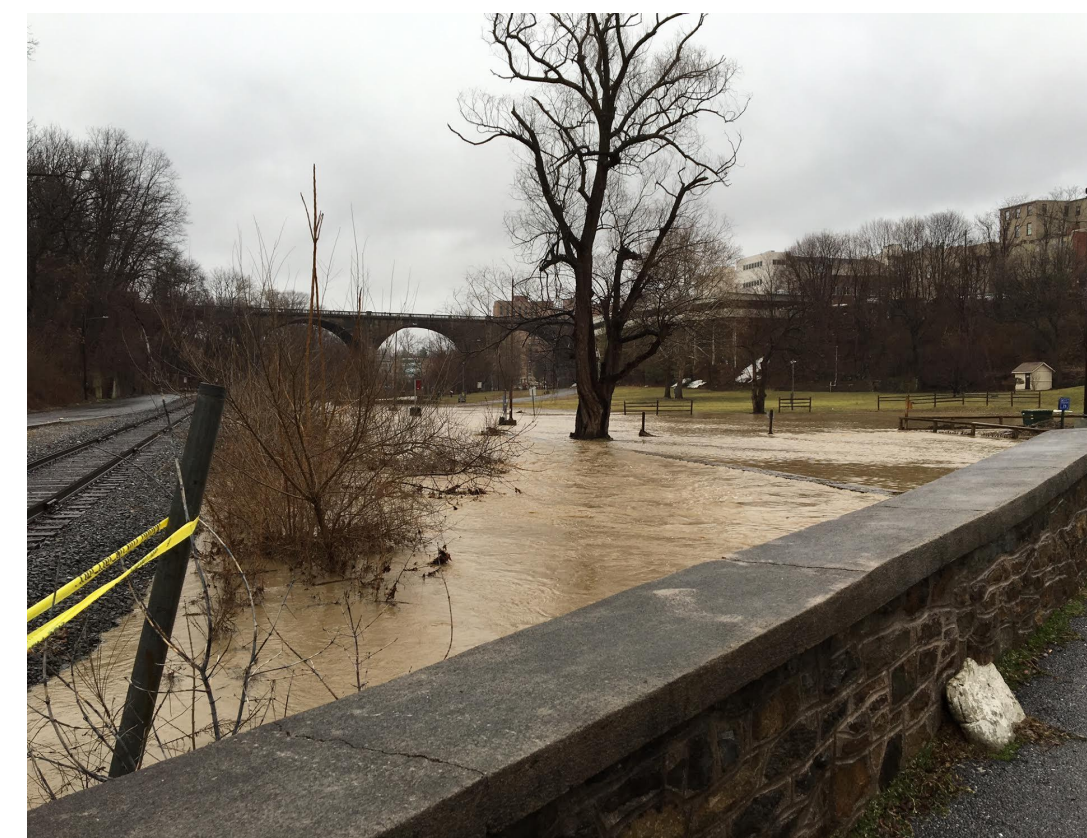
Photo: Flooding of the Monocacy Creek in February 2016 in downtown Bethlehem.
